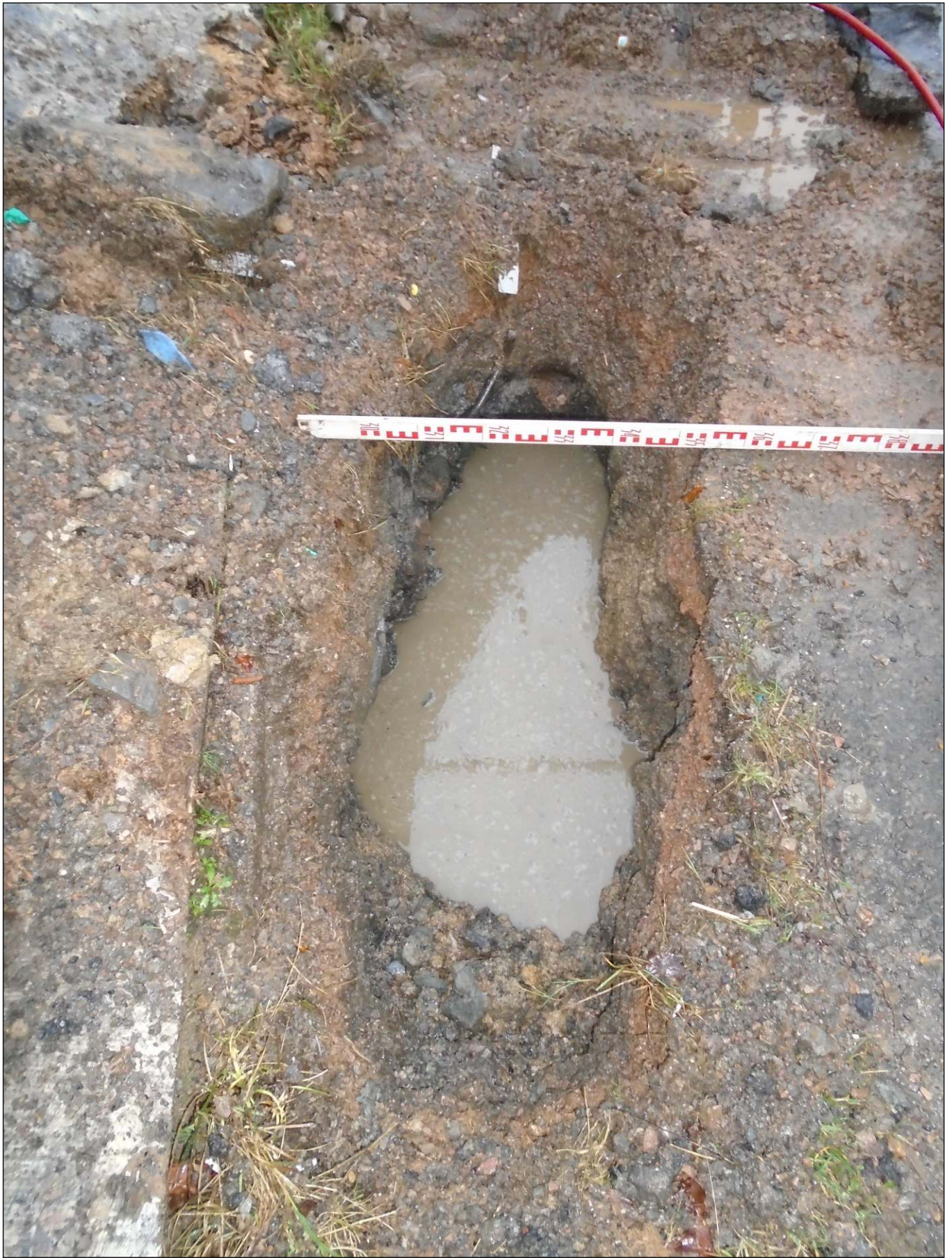
FIGURE 2 BRE365 TEST UNDERWAY AT PENYCOEDCAE.
